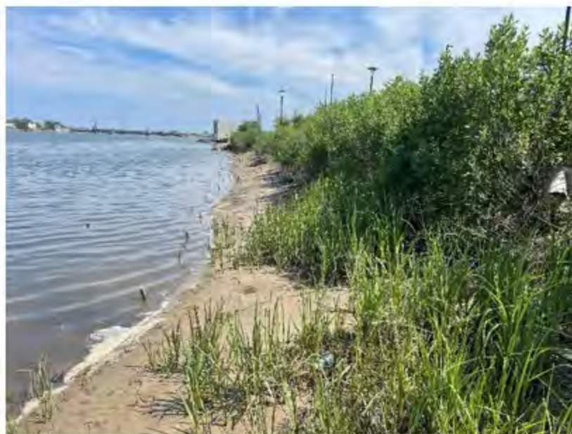
Photo 7. 2025 Stabilized shoreline and planted S. alterniflora getting established.
